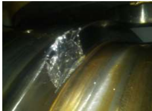
Damaged Barrel Cam
